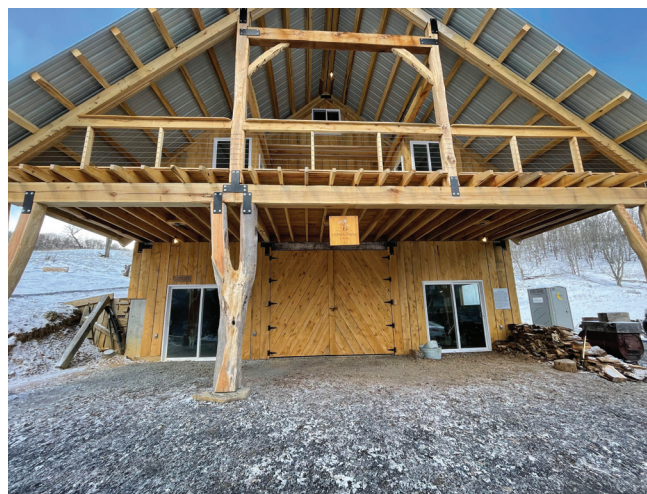
Post and beam sugar house made of locally sourced materials. Downstairs is the sales and storage space, and the evaporator. Upstairs is the office and quarters for a seasonal employee. Photo by Mary Hufford.
